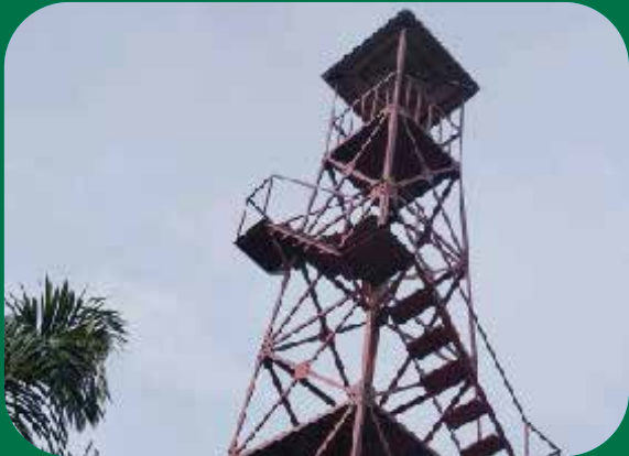
Menara Pantau Api Fire Lookout Tower
